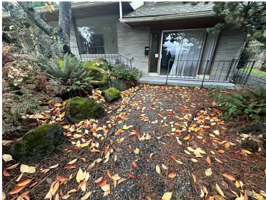
Looking at existing structure and vegetation.
